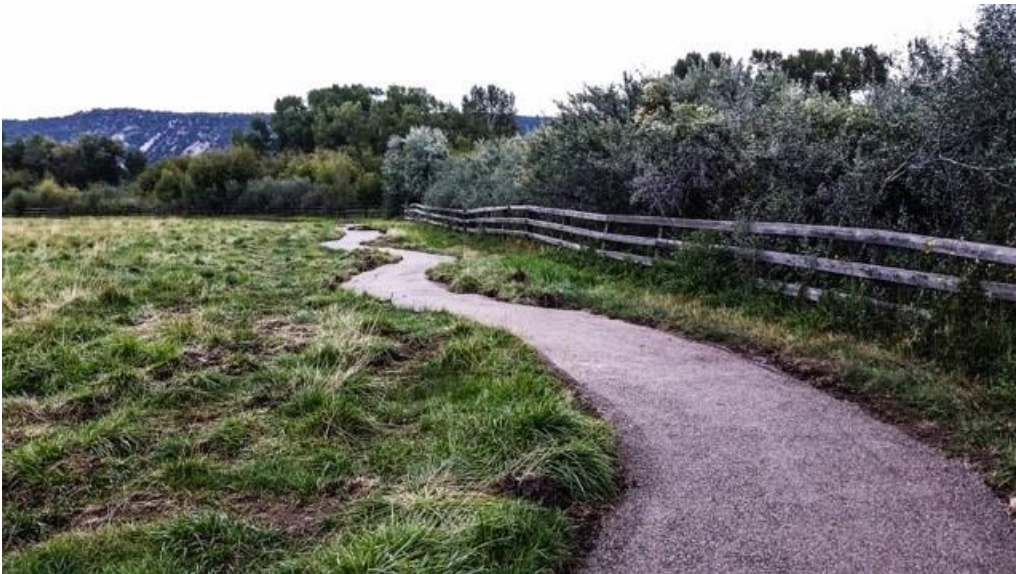
Figure 10. Trail Surfaced with Aggregate Base. (Photo Credit FPC)
