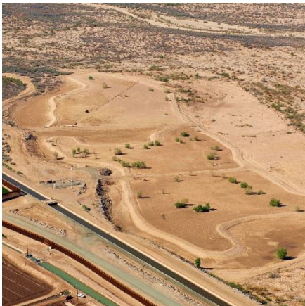
Figure 8. Site Improvements After Land Shaping (Photo Credit FPC)
