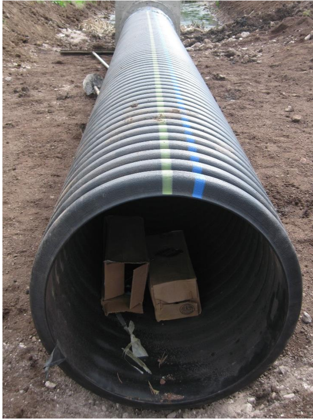
Figure 11. Dual Wall HDPE Culvert Pipe
